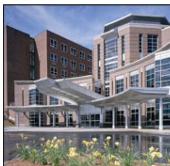
When it came to housing its new 3T MRI, Concord Hospital was seeking a cost-effective and relatively easy solution. The institution worked with PDC Facilities, Inc, and the result has satisfied the radiology department, hospital administrators, and patients.
